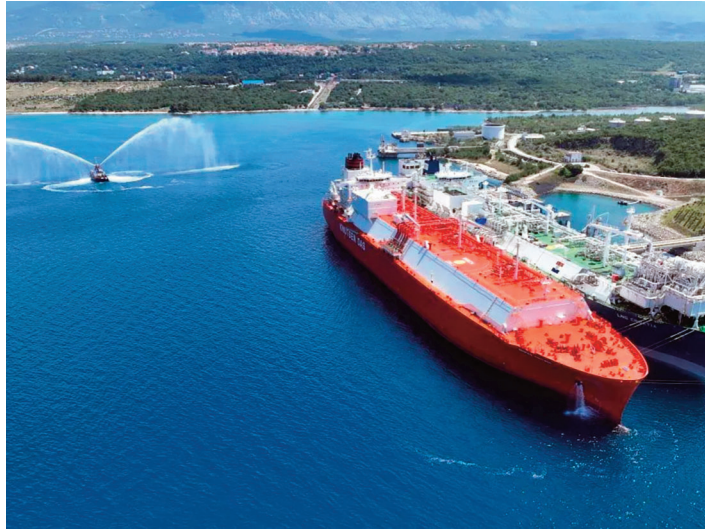
The Krk terminal FSRU is to increase capacity
