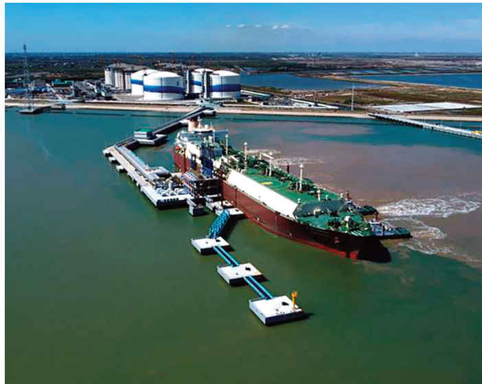
China's Binhai LNG terminal Photo credit: QatarEnergy
